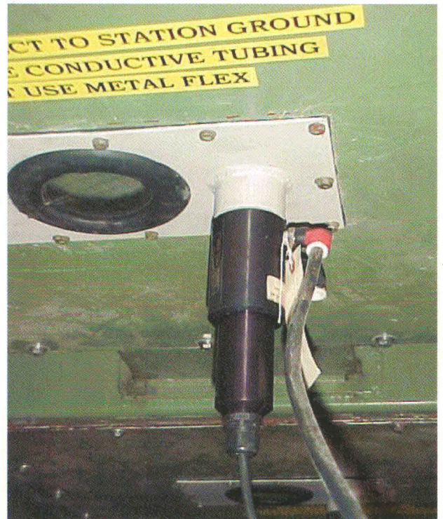
Infra-View® GB/IS Generator Bus Temperature Monitor with air cooling
